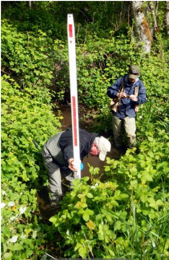
Measuring and recording the gradient of a well-disguised culvert
